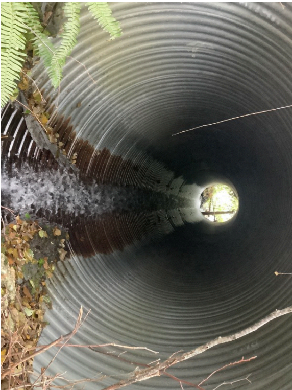
Bush side culvert
