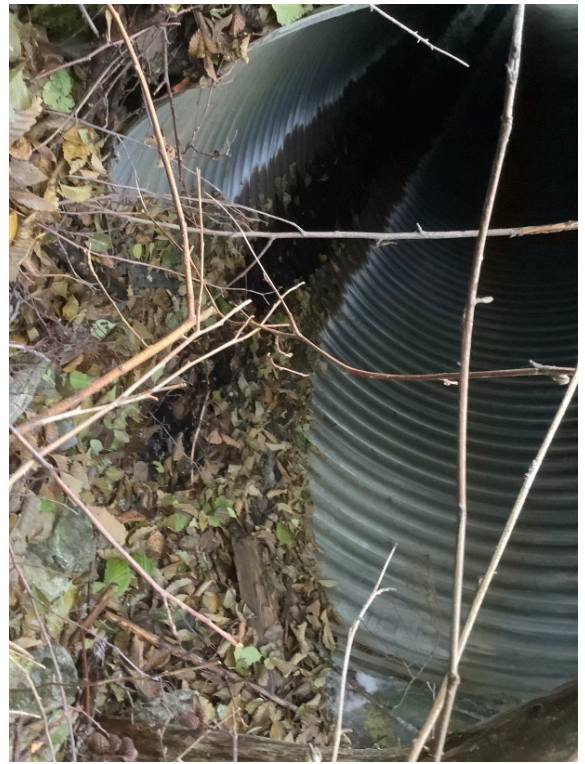
Town side culvert
