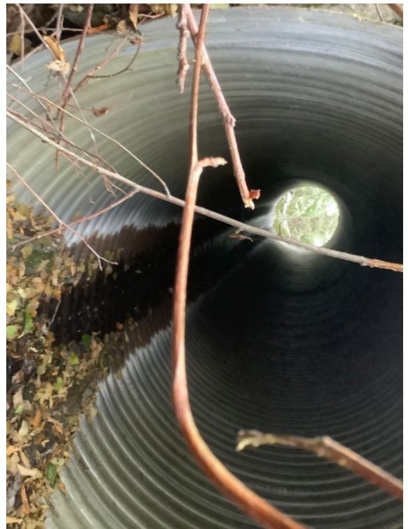
Town side culvert
